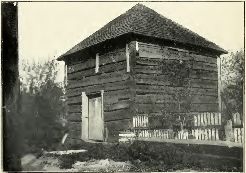
FIRST COURT HOUSE BUILDING FOR GILES COUNTY
